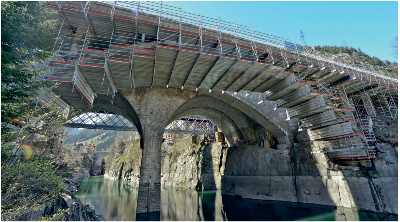
Renovation of a bridge in Göschenen, Switzerland
