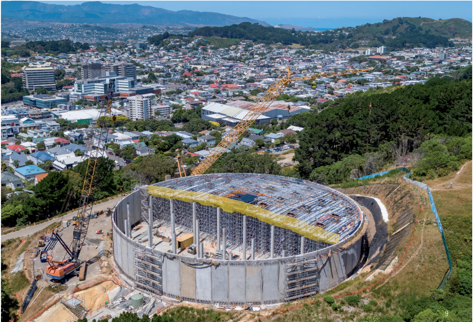
Omāroro Water Reservoir, New Zealand
