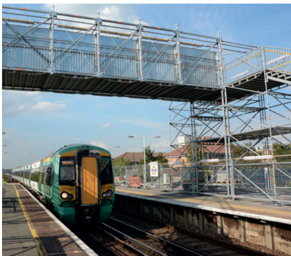
Pedestrian bridge in London, United Kingdom
