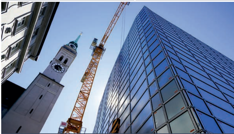
Rebuilding of a city-centre office building, Marienplatz in Munich
