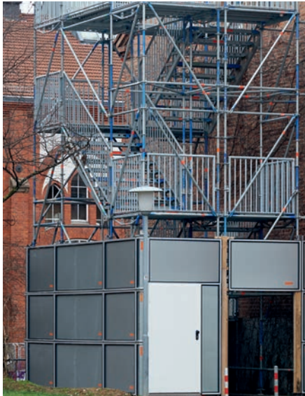
Lockable escape stairtower, Heilbronn
