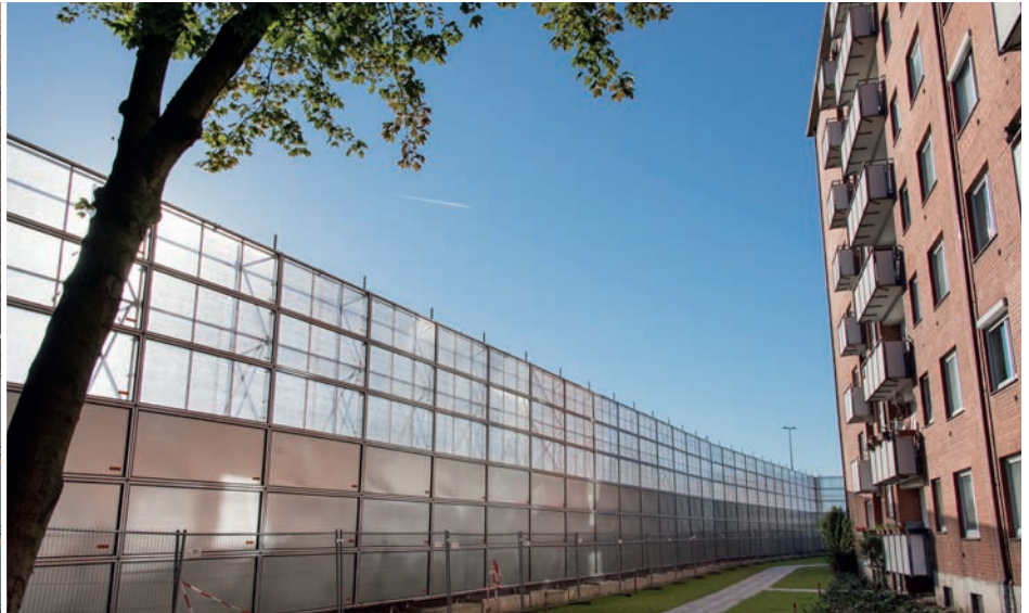
Noise protection wall, Hamburg-Stellingen
