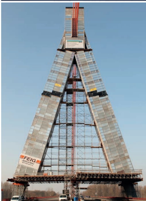
Sandblasting work, Rhine Bridge at Speyer
