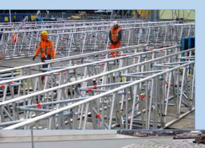
The versatility and strength of the Layher Universal Aluminium (HD) Beam is now a key part of a new manufacturing structure in Newcastle-upon-Tyne where Interlink Scaffolding Ltd. has used the wide roof span to provide a clear working area below. Mark Eddy, Director of Interlink Scaffolding, explains -
