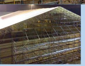
"The Universal Aluminium (HD) Beam's strength allowed bays to be created using sections assembled into 20 metre lengths either side of 18° ridge beam connectors," says Kenneth Redman, Layher's Scottish and Irish Technical Manager. "Keder rails were then fixed to the beams' top chords with translucent Keder sheeting pulled up and over the apex one bay at a time."
