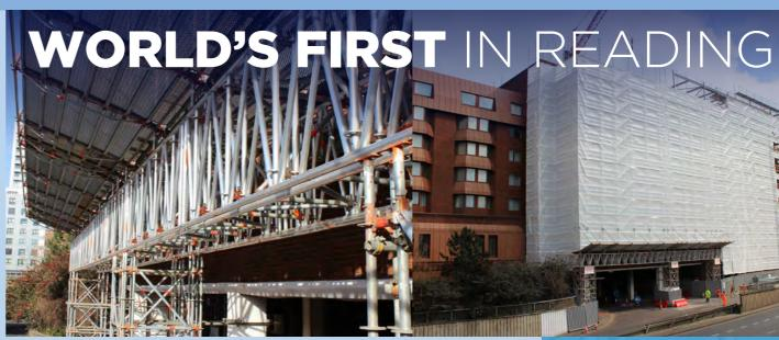
The world's first use of the new HD Beam has centred on the transformation of the old 'Yell House' building for Crown Student Living to become 'Queen's Court'. Archway Services used the beam as a support for the scaffold structure above and to maintain full public access to the on-site car park.
