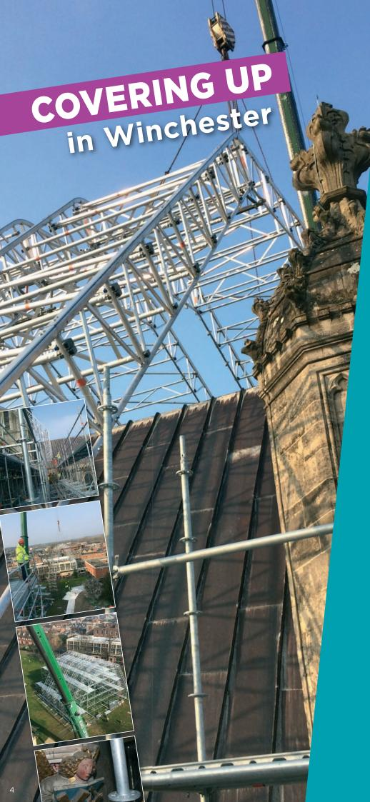
An internationally famous structure, priceless fittings and stonework, and the need for protection for a year – the Layher Allround temporary roof structure that sits over the Presbytery of Winchester Cathedral is impressive by any measure. Installed by Blencowe Scaffolding, the roof build is part of a four-year restoration programme and has directly answered many specific questions raised at the site –
