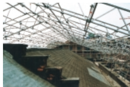
The Layher Keder roof system has brought tangible benefits to the refurbishment of Murrays' Mills in Manchester.
