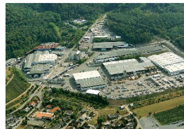
The Layher Head Office and factory in Germany
