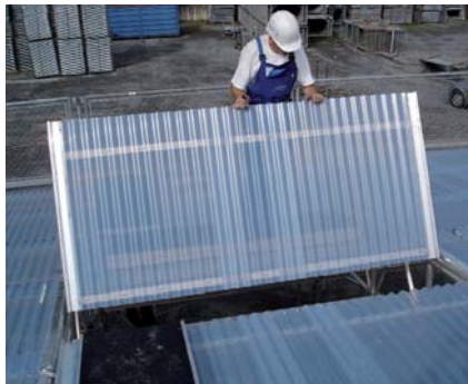
The new, patented light weight cassette roof system provides effective protection and is simple and easy to handle
