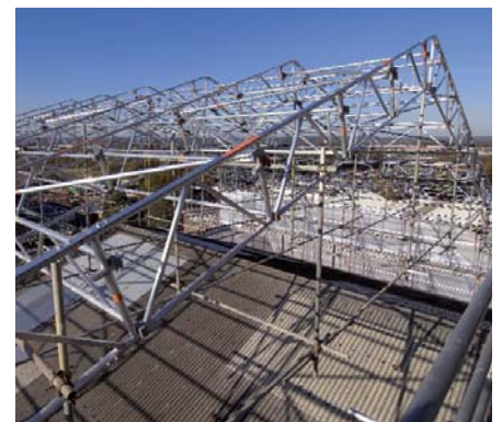
The internal load bearing birdcage structure that provides back-propping (above right)
