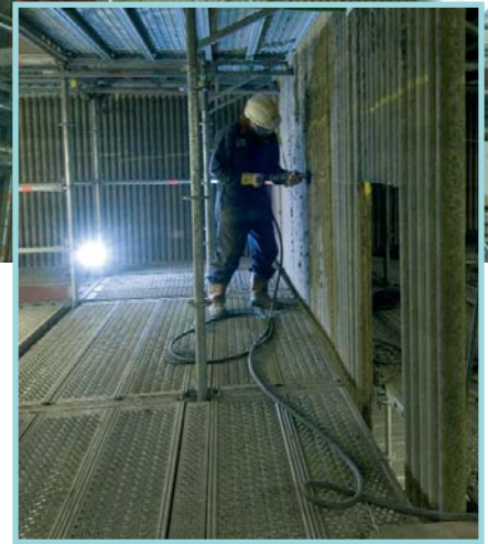
Layher Scaffolding has helped work at Drax – including cutting and replacing boiler wall tubes (right).
