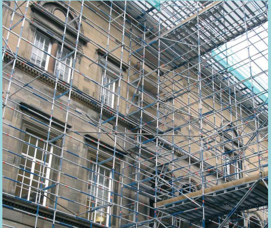
Clear access with Allround® scaffolding at Edinburgh University.
