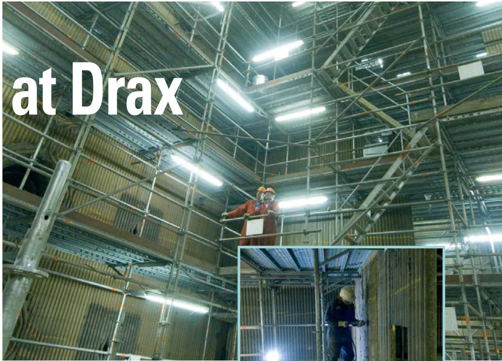
Layher Scaffolding has helped work at Drax – including cutting and replacing boiler wall tubes (right).
